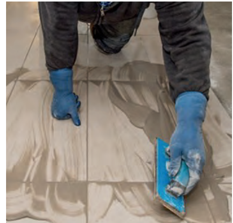
Figure 2 - Cement grout application
