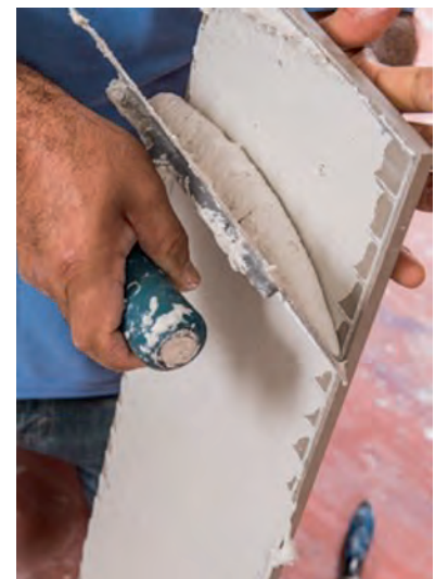
Figure 1 - Back-buttering (flat-back troweling)
