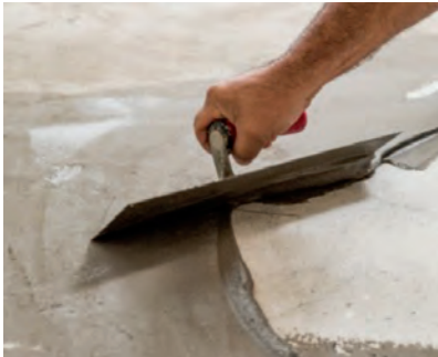
Figure 5 - Applying patch to concrete substrate
