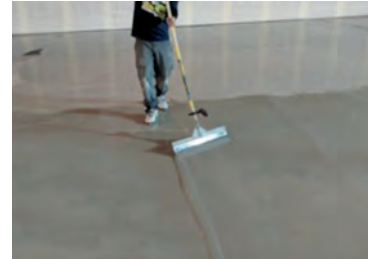
Figure 6 - Pouring self-leveling underlayment
