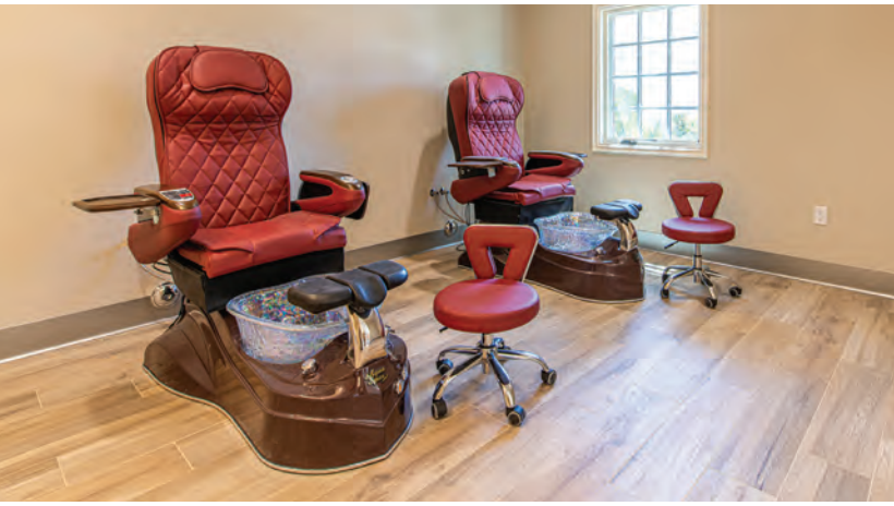
Care center -LHT porcelain plank tile installed with Merkrete 720 DUSTLESS LHT Mortar and Duracolor Grout.
