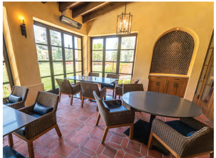
Bar & grill seating area installed with Merkrete Hydro Guard SP-1, 735 DUSTLESS Premium Flex and Pro Epoxy Grout.
