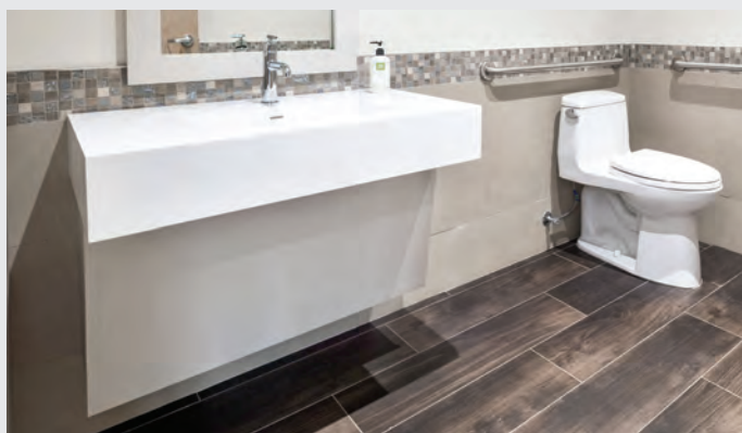
Restroom installed with Merkrete 820 DUSTLESS Merlite on walls with Duracolor Grout.
