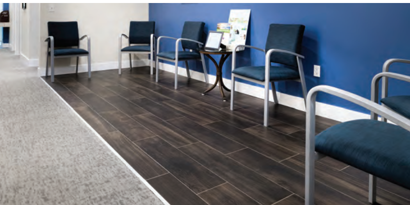
Patient Waiting Area: LHT porcelain plank tile and commercial carpet squares installed with SikaBond®-150 Premium Floor Adhesive.
