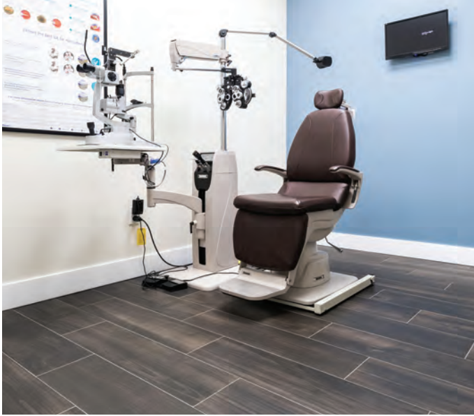
Procedure suite: LHT porcelain plank tile installed with Merkrete 720 DUSTLESS LHT Mortar and Duracolor Grout.
