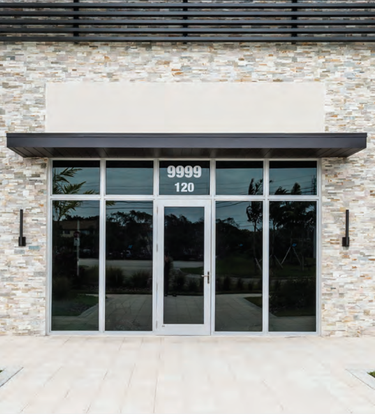
Natural Stone installed with Hydro Guard SP1 and Merkrete 820 DUSTLESS Merlite.
