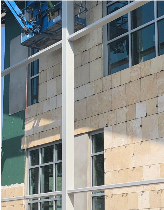
Exterior protected using Merkrete's Hydro Guard SP-1 waterproofing & crack isolation membrane.
