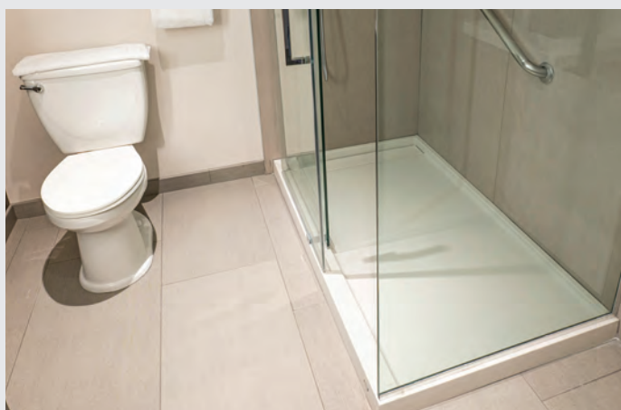
Merkrete's Hydro Guard SP-1 waterproofs Sheraton's 490 guest bathrooms.
